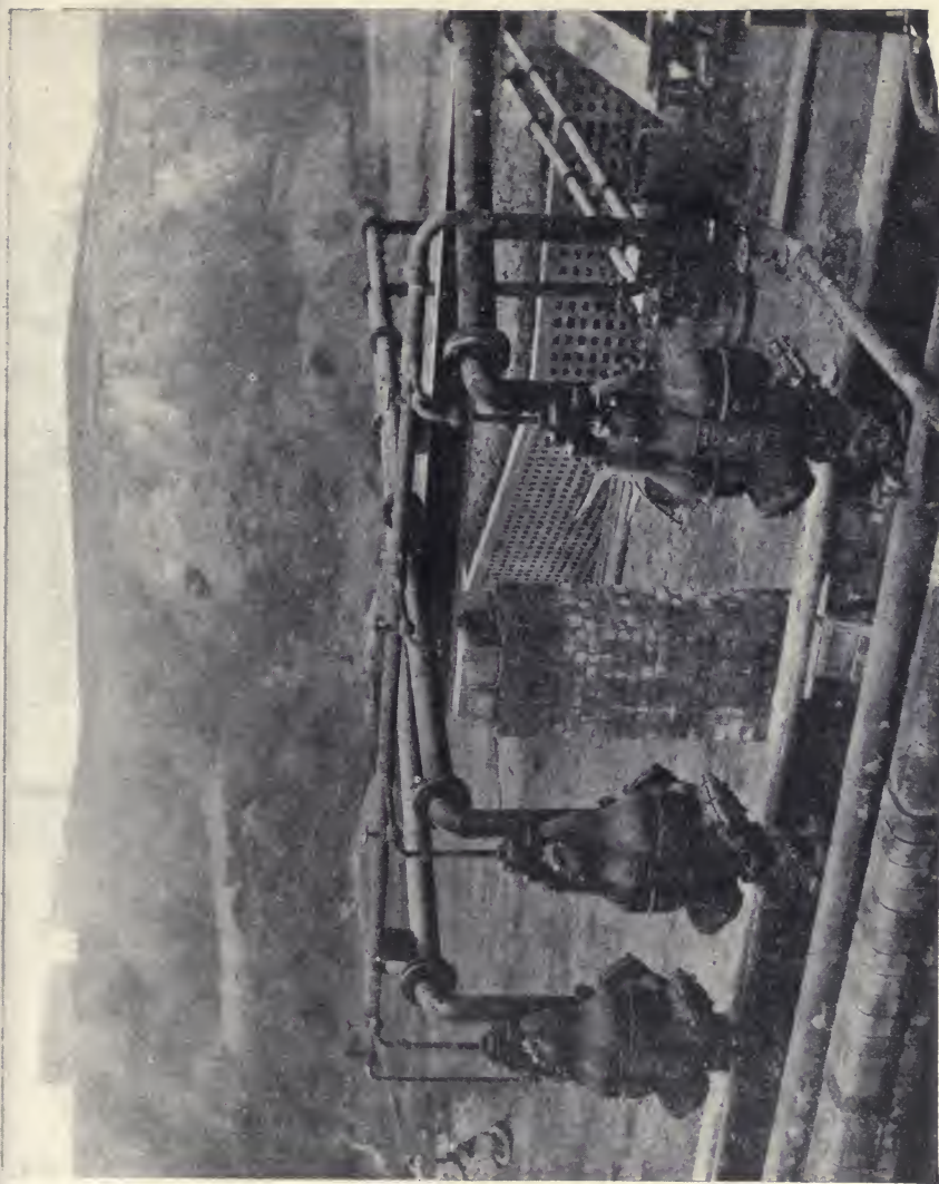
Fig. 38A. Application of Pulsometer Pump to Sprinklers.
